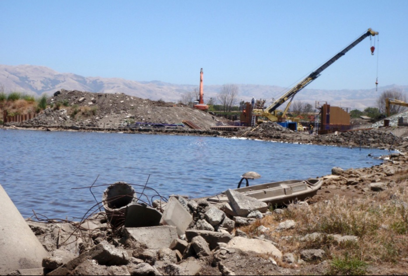
A8 Notch Construction
